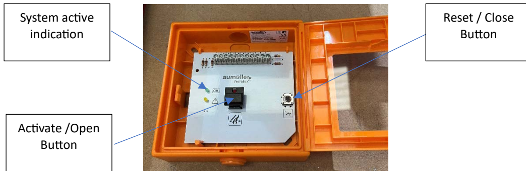
Picture 2 – Manual Call Point (aka Breakglass Unit)
